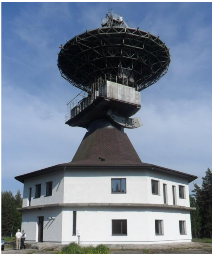
Figure 3 ~ RT-16 in Irbene near Ventspils, Latvia. The basement contains a workshop, the control center, sleeping rooms, a kitchen, a living room, offices and a restroom.
